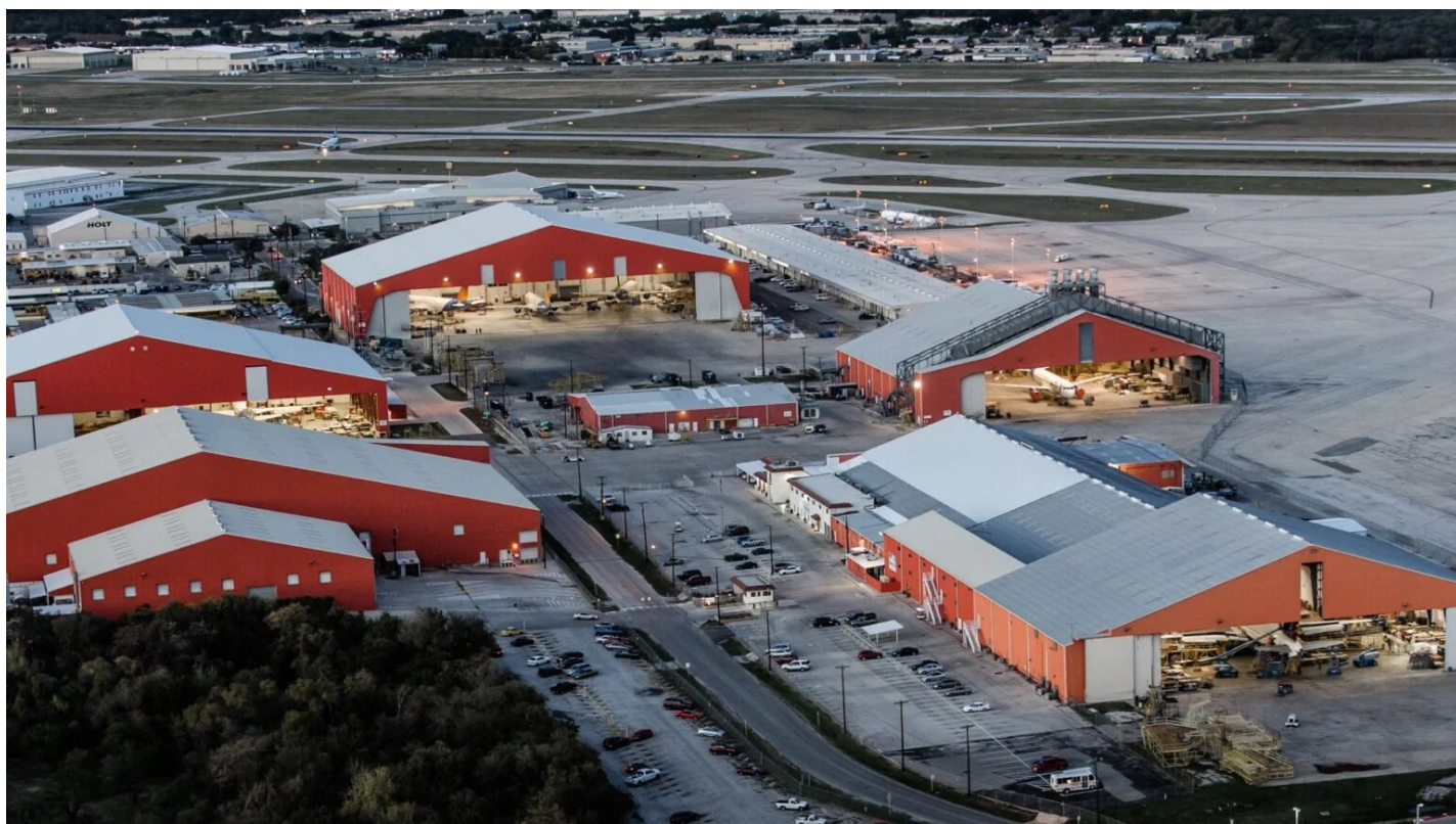
The ST Engineering maintenance, repair and overhaul facility in San Antonio, Texas, includes a hangar for cargo conversions (right foreground). ST Engineering will suspend conversion work there by the end of the year. (Photo: ST Engineering)
